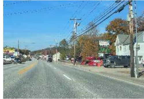
Figure 19: Utility poles reducing effective sidewalk width
